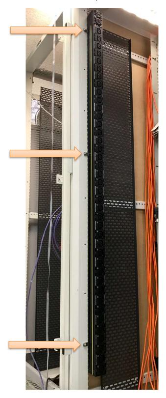
N.B. The VPB should be earthed for safety reasons to avoid electric shock hazards. You may fit the VPB panel sideways also facing inwards to the back the units or outwards facing away from the units.
