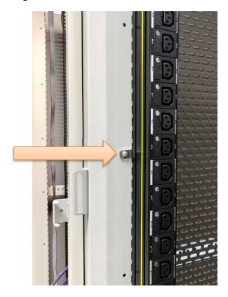
7. Fit the third mounting bracket with M5 nut and bold.
